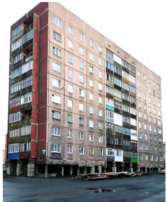
The elevation of buildings (and other infrastructure) onto pillars allows for a ventilated layer between the structure and the ground, which helps protect against permafrost degradation: Norilsk, Russia. Photo: Nadezhda Zamyatina/reprinted from ECONOR 2020.
