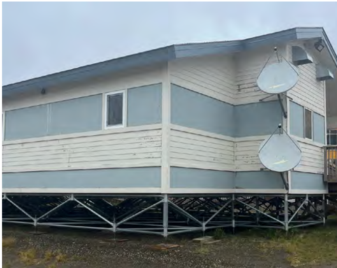
Light structures are built on top of adjustable frame foundations placed directly on top of the ground, Nome. Photo: Maryana Shnitser
