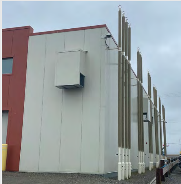
Thermosyphons are installed at the side of the building to provide additional cooling to permafrost under the buildings. Ventilated crawl spaces designed to protect permafrost from heat from the building above, as they limit snow accumulation in the winter and provide shade in the summer, Nome. Photo: Maryana Shnitser.
