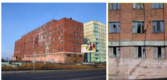
Building damaged by permafrost degradation, Norilsk, Russia. (Photo from 2013, now the building is dismantled). Photo: Nadezhda Zamyatina/reprinted from ECONOR 2020 Detail of façade: Building damaged by permafrost degradation, Norilsk, Russia. (Photo from 2013, now the building is dismantled). Photo: Nadezhda Zamyatina/reprinted from ECONOR 2020.
