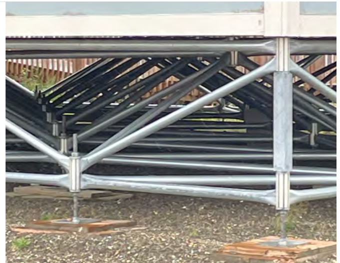
Light structures are built on top of adjustable frame foundations placed directly on top of the ground, Nome. Photo: Maryana Shnitser
