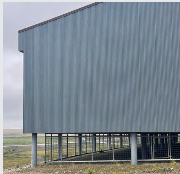
Thermosyphons are installed at the side of the building to provide additional cooling to permafrost under the buildings. Ventilated crawl spaces designed to protect permafrost from heat from the building above, as they limit snow accumulation in the winter and provide shade in the summer, Nome. Photo: Maryana Shnitser.
